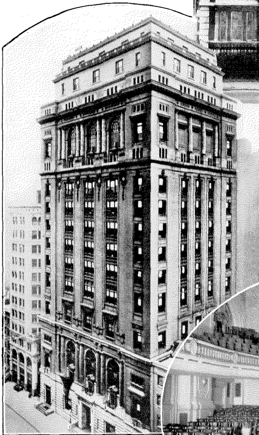
The Engineering Societies Building, in which the Headquarters of the American Institute of Electrical Engineers are located and in which New York City Meetings are held.
